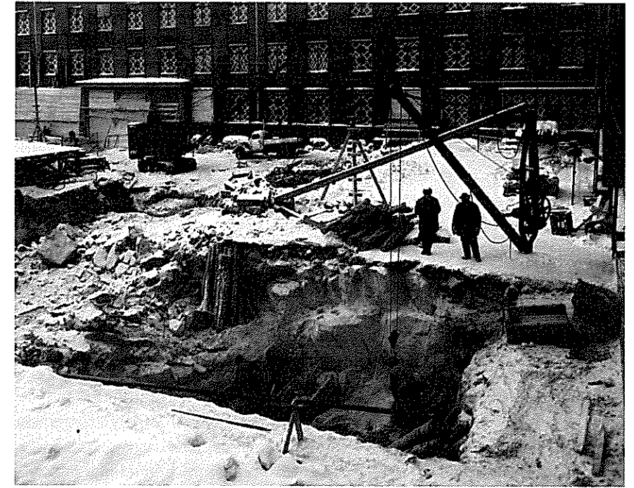
shelter Constructing a bomb shelter, 8th April 1940, HCM, photo Roos
